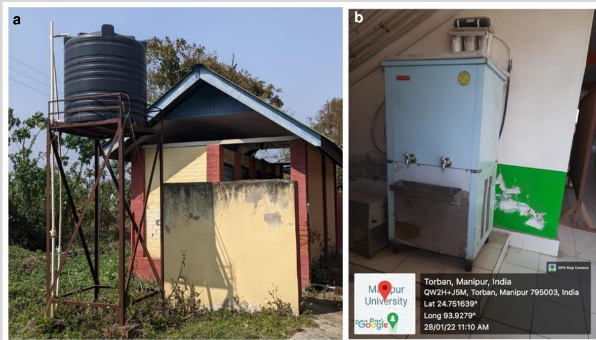
Photograph Plate 7: a. the water-supply-system to the Washrooms and the departments installed with polycan; and b. the drinking water facility installed in the department.
